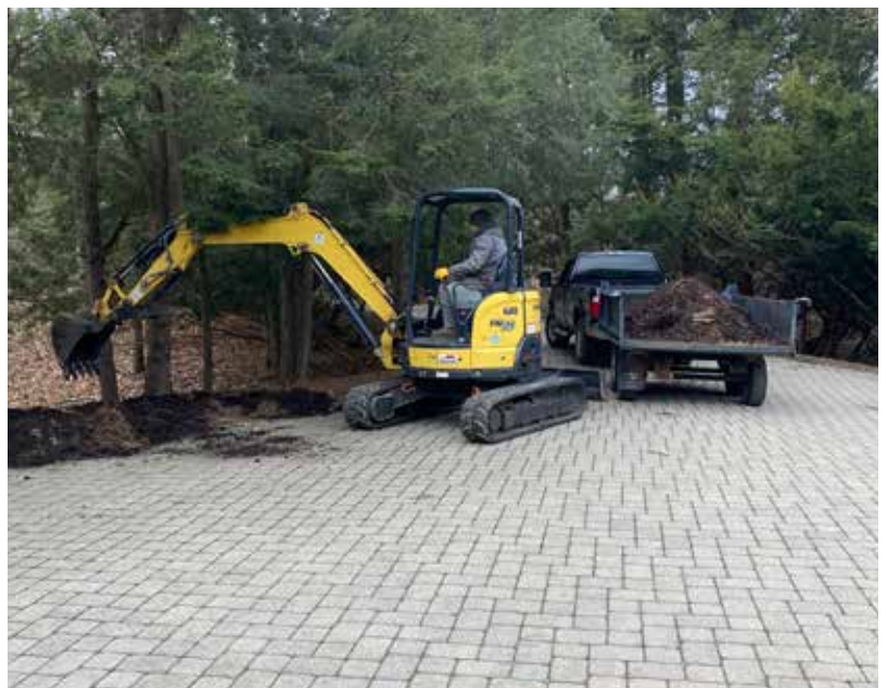
Altering the grade to allow better waterflow
